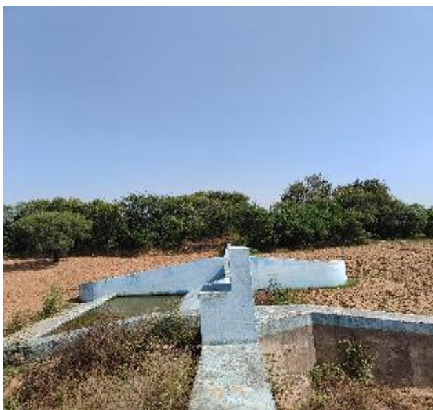
Figure 10: Check Dam/Nala Bund built at Guwara village
