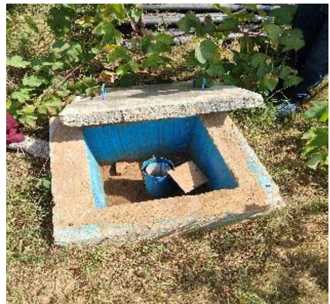
Figure 11: Piezometer installed at Guwara Village
